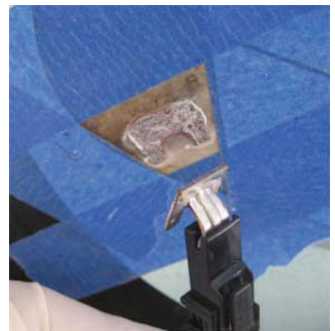
Mask off damaged area
